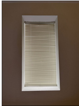
The skylight is covered with blinds and could not be inspected
