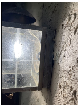
Caulk around the exterior light fixtures.
