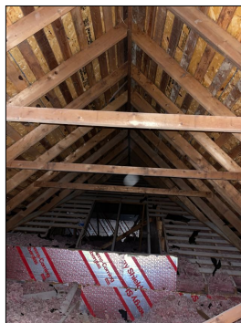
RAFTER COLLAR TIES ARE PRESENT!
