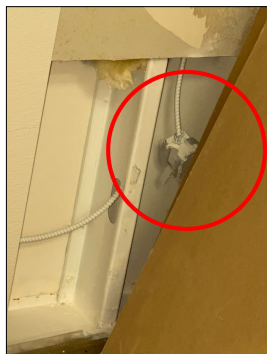
Hanging junction box: West boarding 2nd room from south NW corner
