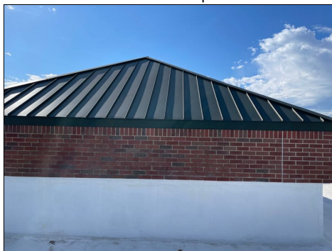
Metal standing seam roofing noted. Over front center area.
