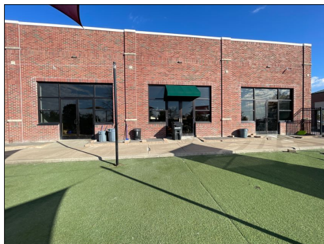
Commercial Grade Metal Double Doors with GLASS: 3- Sets on the South side of the building.
