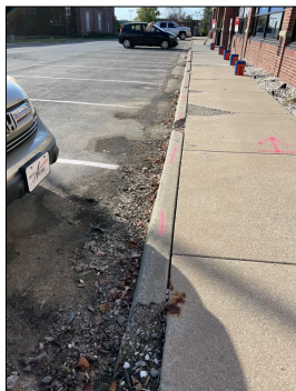
Poured Concrete Curb At front sidewalk area.
